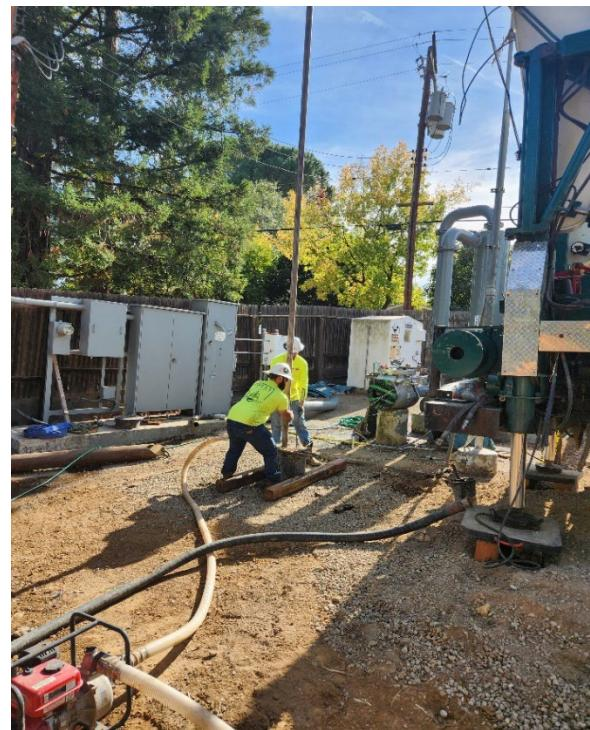
Ladera ASR Well Project: The existing well was destroyed on September 27, 2024. The contractor has set up a sound wall and has installed the casing for the new well. The new well has been drilled to a depth of approximately 520 feet and is currently being developed. Pictures below show the sound wall and conductor casing installed.
