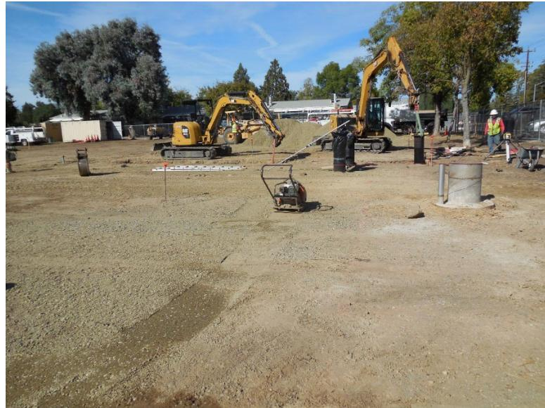
Winding Way ASR Well Project: The District staff has coordinated with SMUD to temporarily remove the power line and connection to the District owned residential home on Charleston Way in order to facilitate the access of high profile equipment into the project site. The existing well was destroyed on November 5, 2024 and the sound wall used for the drilling of the new well is currently being installed. See photos below for the preparation of existing well destruction.
