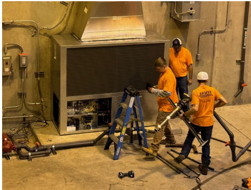
Raw Water Pump Room HVAC Replacement
