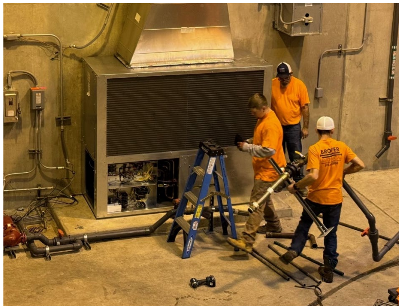
Raw Water Pump Room HVAC Replacement
