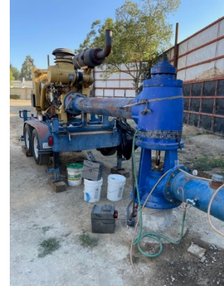
Photo - Developing the new La Sierra ASR well using step pumping at different flow rates. (August 2023)
