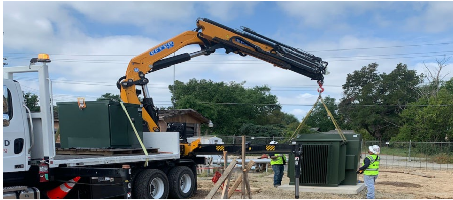
SMUD setting new transformer at the La Vista Tank site
