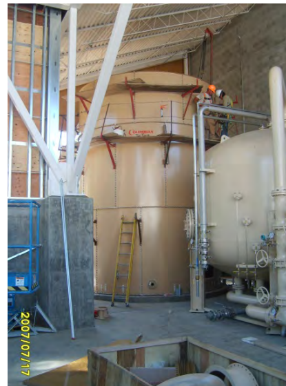
Construction of GET LB GAC Filters and Backwash Tank
