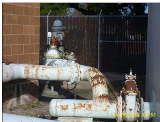
La Vista Well and Tank: Aging Outlet Piping
