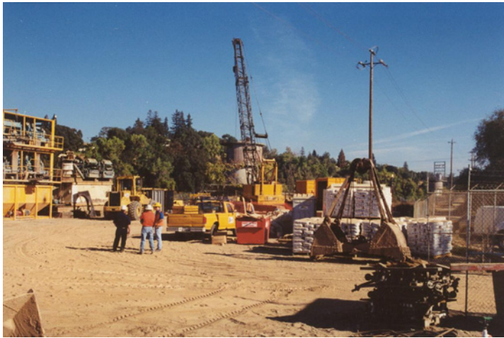
American River Microtunnel Crossing – 48-inch Diameter Pipe – photograph courtesy of Peggy Berry, District Resident
