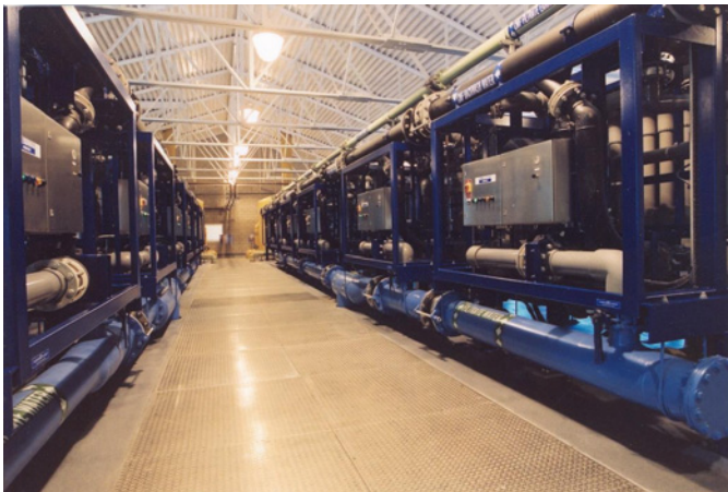
Bajamont Membrane Filtration Process Equipment – photograph courtesy of Peggy Berry, District Resident
