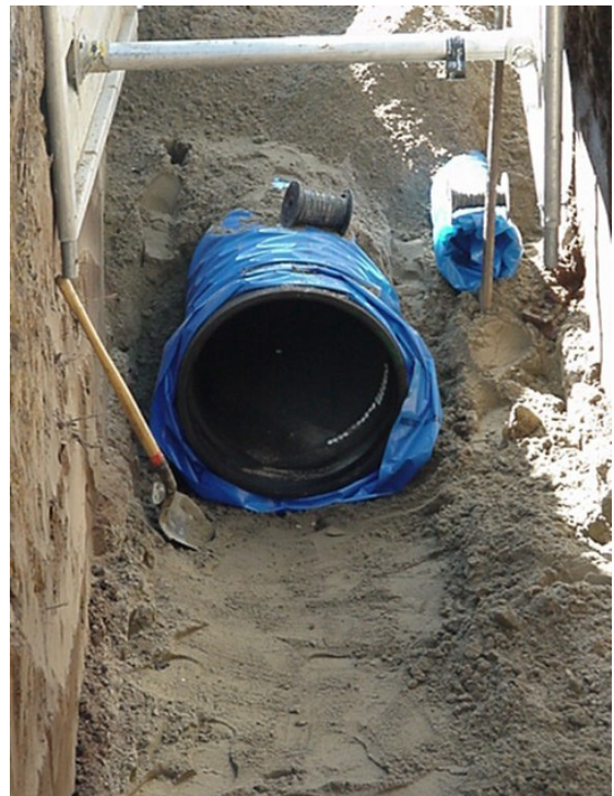
24-inch transmission main (left) with 8-inch distribution main (right) in common trench.
