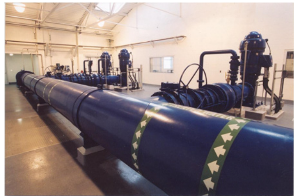
Bajamont WTP Clearwell Treated Water Pumps
