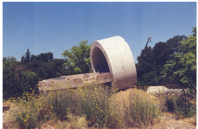
Removal of Above Ground Portion of Ranney Collector in Progress
