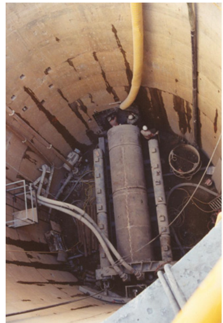
American River Crossing – Microtunnel Shaft
