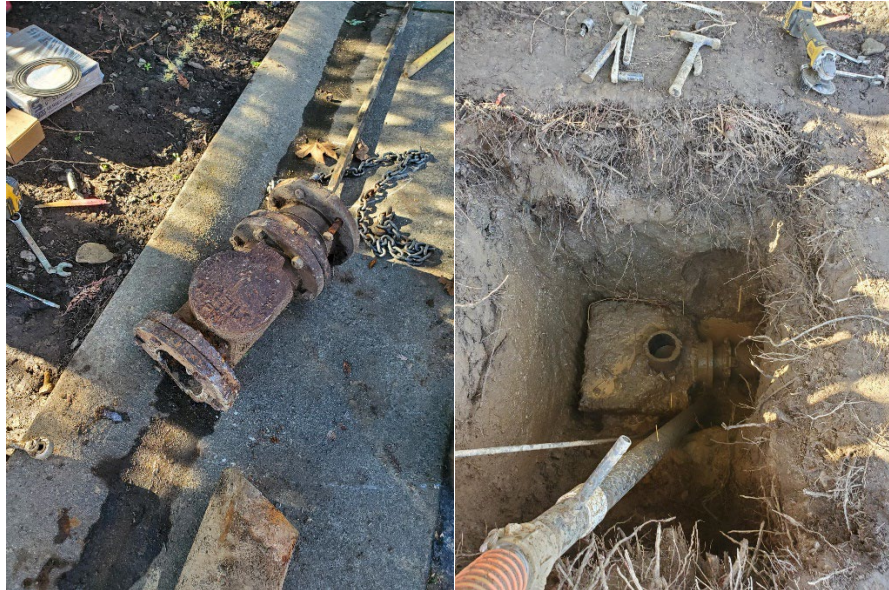
La Sendita Ln. Hit hydrant bury replacement due to faulty check valve.
