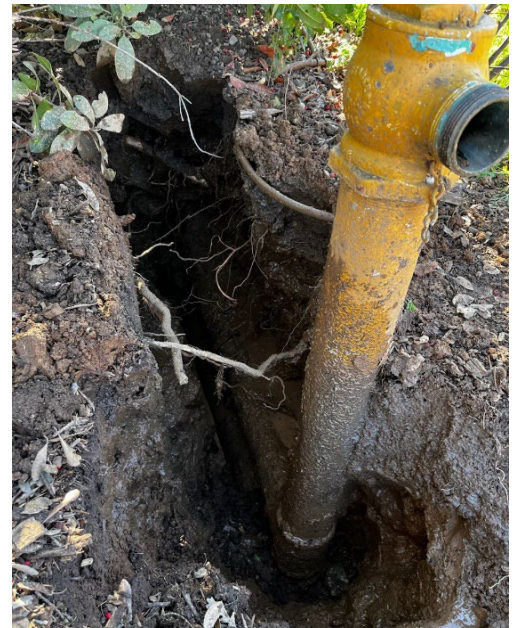
4-inch steel main with wharf hydrant
