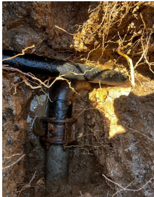
4-inch steel main with wharf hydrant
