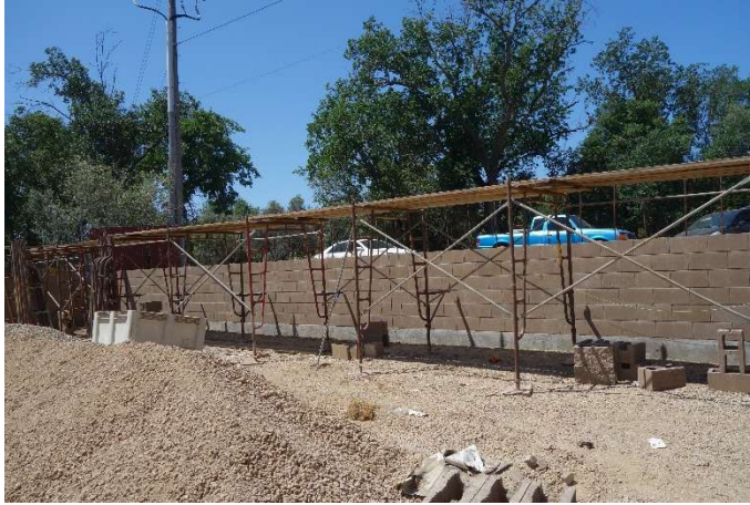
East CMU Wall adjacent new tank
