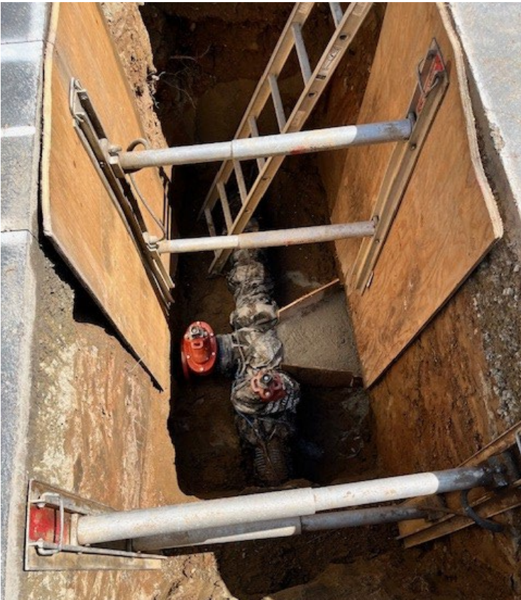
8" T with Butterfly Valves and Thrust Block
