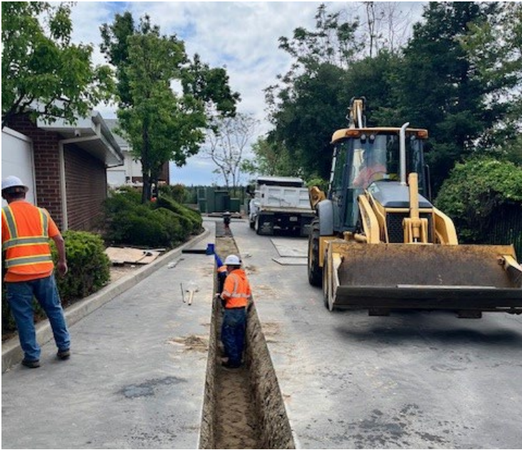
Distribution Crew Installing New Hydrant Main
