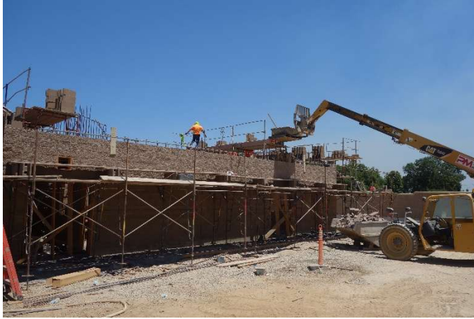
Booster Pump Station Blockwork
