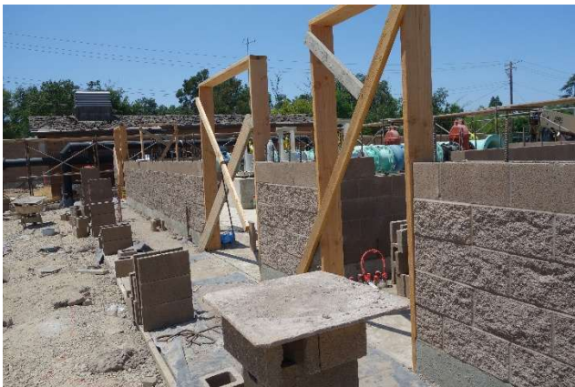
Booster Pump Station Blockwork
