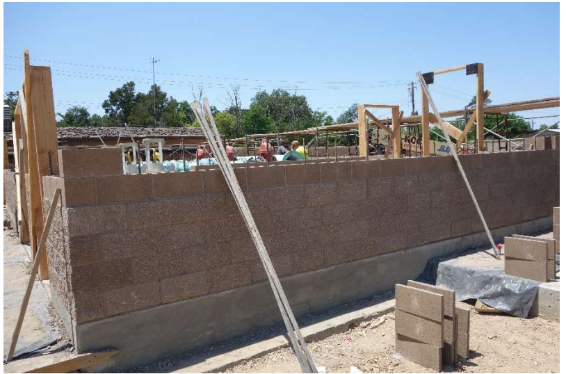
Booster Pump Station Blockwork
