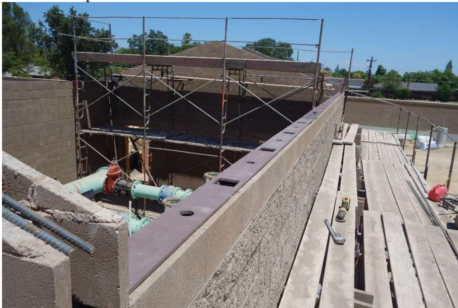
Booster Pump Station Embeds
