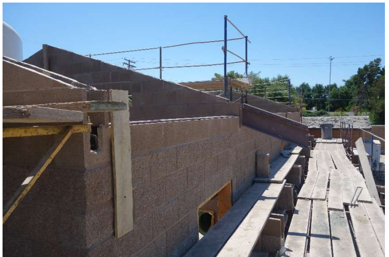
Booster Pump Station Blockwork
