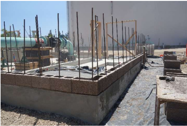
Booster Pump Station Commence Blockwork
