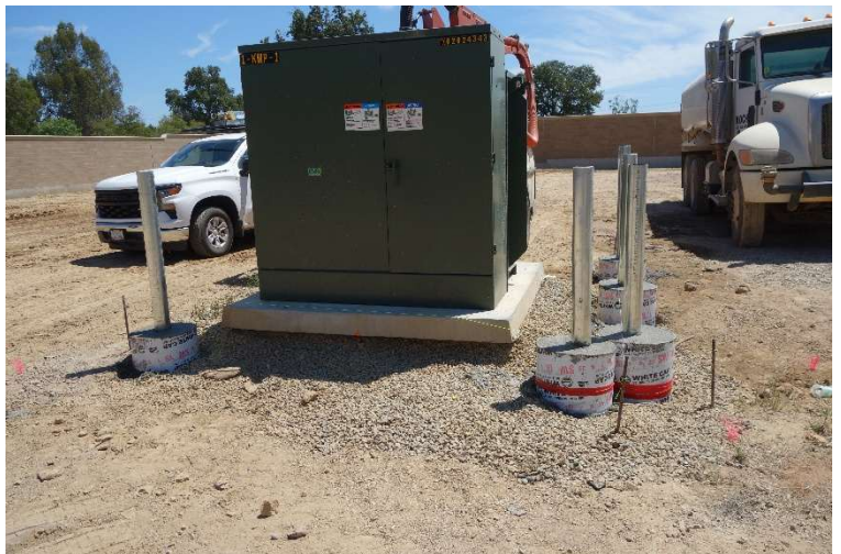
Bollard installation
