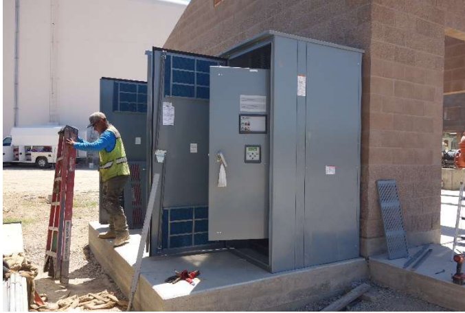
Switchgear Installation
