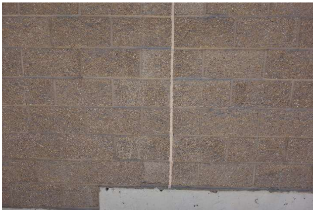
Caulking at CMU joints
