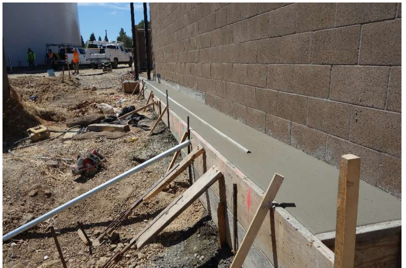
Sliding Gate concrete
