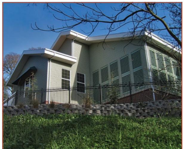
*Architectural features that allow the plant to blend with the neighborhood include brick veneer, retaining walls, and acoustical louvers.*
